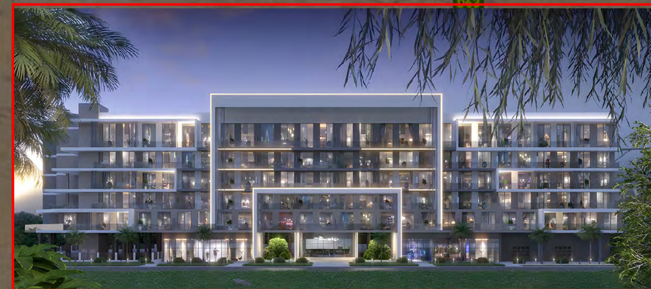
LAYA COURTYARD DUBAI STUDIO CITY, UAE
